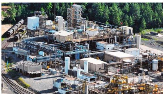
LANXESS's Emerald Innovation 3000 flame retardant production unit in El Dorado, Arkansas, USA. The debottlenecking project increases the output from 10,000 to 14,000 MT per year. Photo: LANXESS AG
